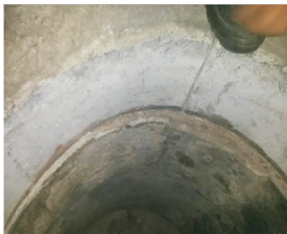
Figure H Ledge between the coil grout and the upper ring
